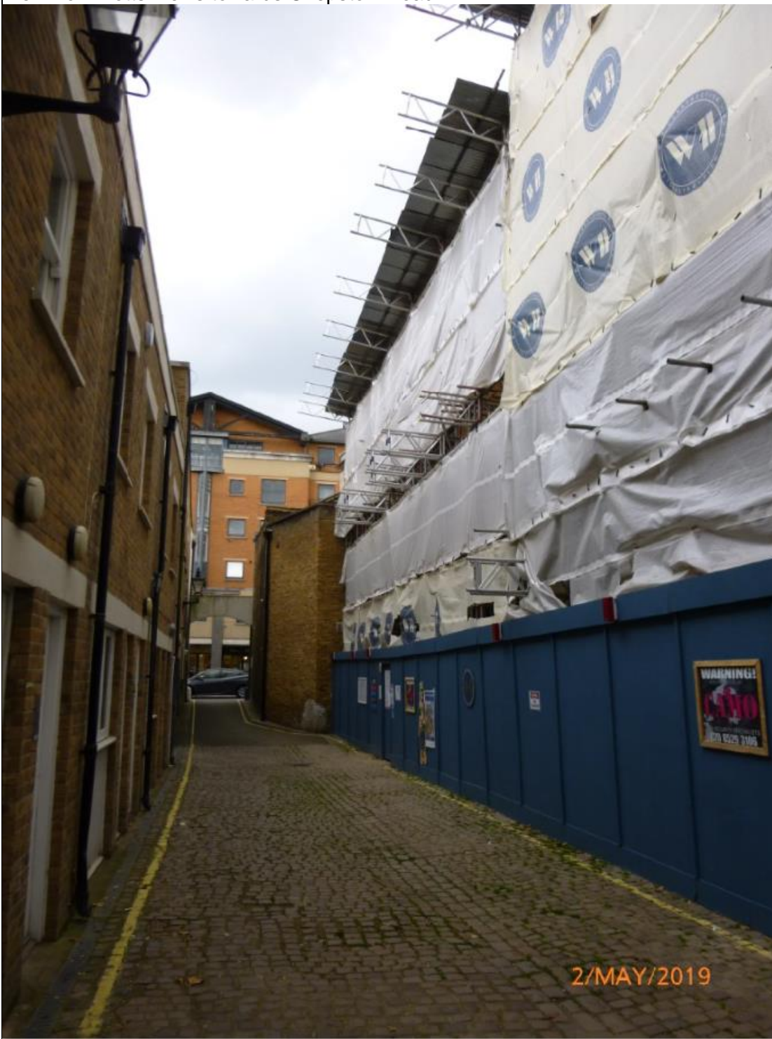
View from Botts Mews towards Chepstow Road
